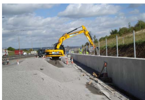
Figure 27 – The use of bottom ash (left) as road base for road construction e.g. the M25 in the UK (right)
