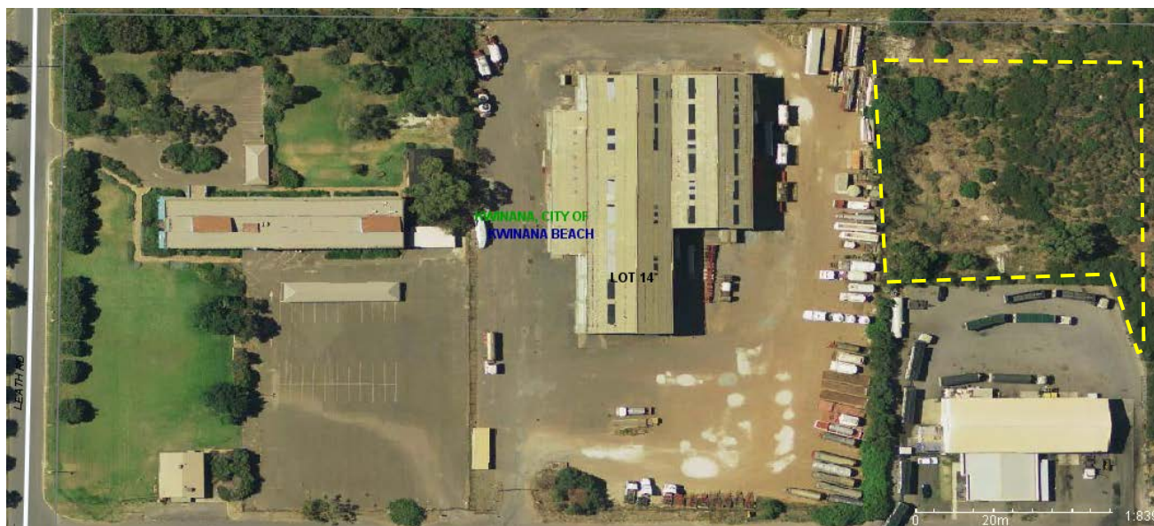
Figure 66 – Photo of the proposed site on Lot 14 highlighting the area of vegetation expected to be cleared under the proposal
